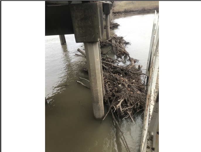
Span 10-11 drift
